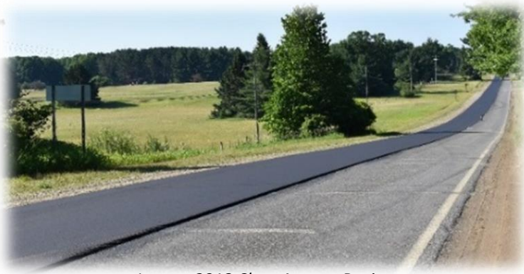
Image: 2018 Clare Avenue Paving
