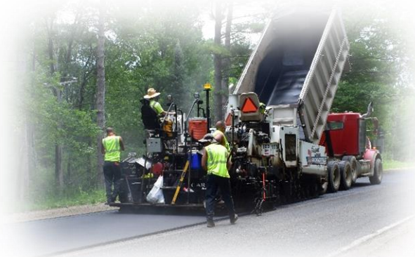
Image: 2018 Clare Avenue Paving
